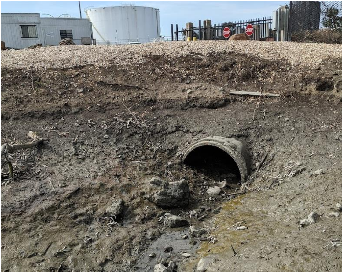
Figure 5. Stormwater outfall that crosses wall alignment and is inundated at high tide.
